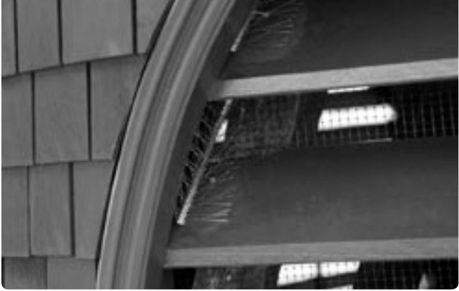
A DETAIL OF LVPC'S NEWLY RESTORED STEEPLE.
